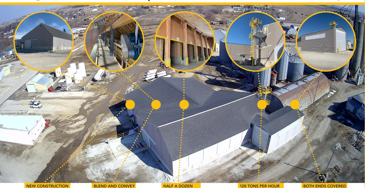
This project was a new-from-the-groundup dry fertilizer shed for the cooperative, and its first season in use will be this spring. The site's handling equipment includes Doyle products such as receiving equipment, two vertical blenders and loadout conveyors.
