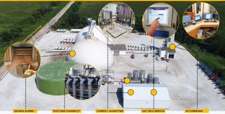
The domes have capacity for 120 railcars of fertilizer each. Bulk head openings allow for payloader access to feed the in-ground Ranco pit. There's room to expand with two more domes.
