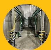
The anhydrous setup includes 30,000-gal. and 20,000-gal. stationary tanks.
