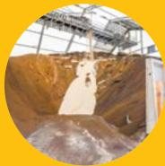
The building is loaded by both trucks and rail cars. The fertilizer storage bins were formed using precast concrete walls.
